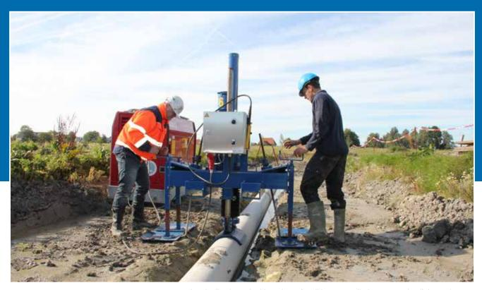
The pipeline is pushed into the soft soil in a controlled manner using light equipment.
