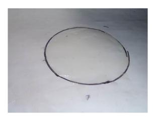
After preparing the hull area, place the transducer and nut in the proposed position and draw around the outside of the nut to give you a guide.
