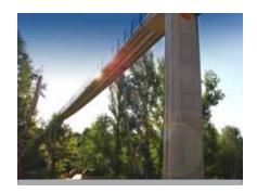
The world's longest stress ribbon bridge was awarded the JEC Innovation Award 2012 in the construction category. Future Fibres provided wound, unidirectional solid carbon fibre cables as the primary loadbearing supports of this footbridge built in Cuenca, Spain.
