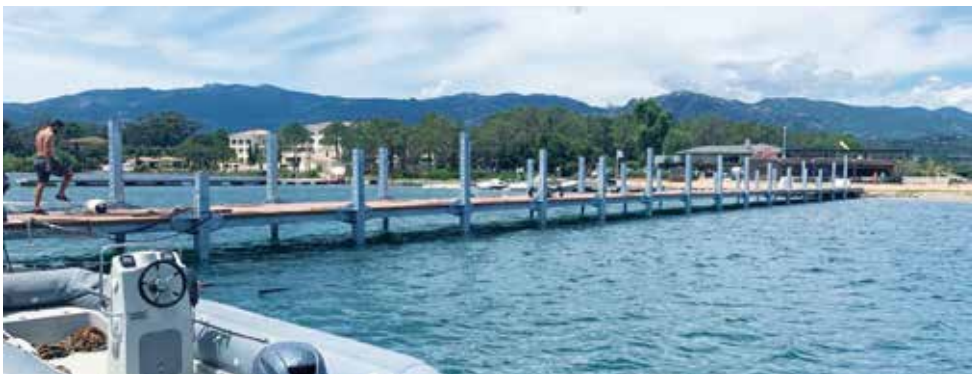
Prefabricated, fixed pontoon, seasonal, Porto Vecchio Marine, Porto Vecchio - France
