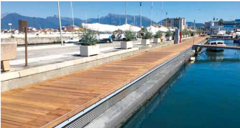
Renovation of a fixed quay, La Maddonnina, Viareggio - Italy
