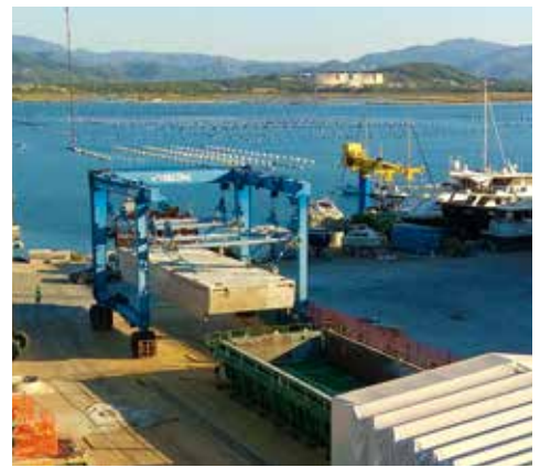
Mobile site for construction of breakwater elements 20x6m, Olbia - Italy
