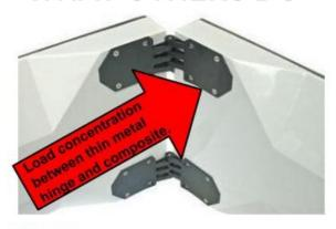
**Hinges:** separate metal parts, attached to the main structure.
