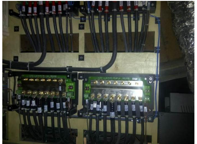
Navylec Power distribution example
